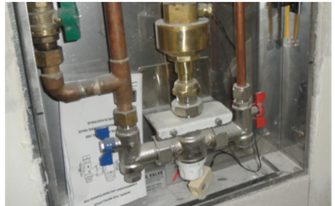
Image 2 – TMV Monitoring system typical installation.
